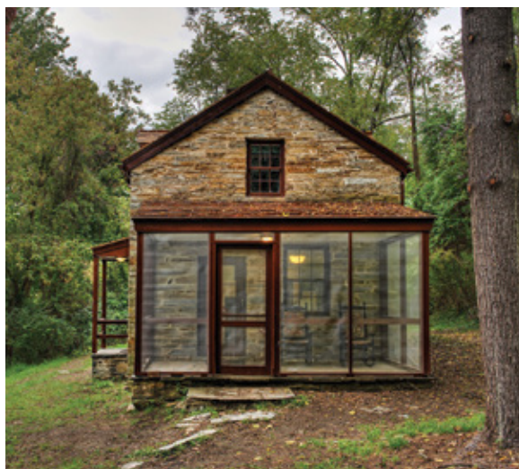
Forty or so lockhouses still stand along the Canal, a few of which have been restored to accommodate overnight guests.
